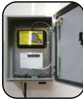
Sea Marshall Base Unit and auto dialer installed in a enclosure
